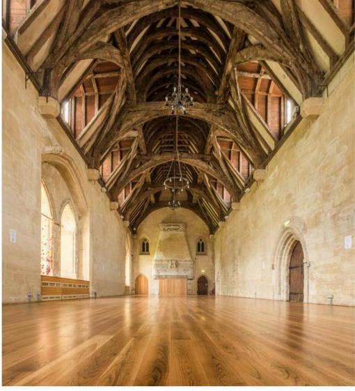
The roof was installed between the inner and outer walls which were relined with ashlar but its length necessitated the demolition of part of the outer curtain wall at the eastern end of the hall. Both fireplaces are French dating from the 15th Century, the more striking of the two is at the west end.
